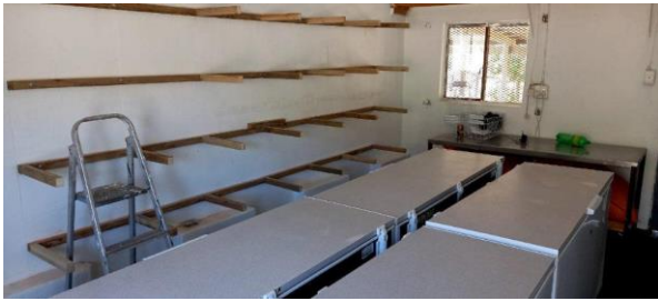
Above, preparing the storeroom
